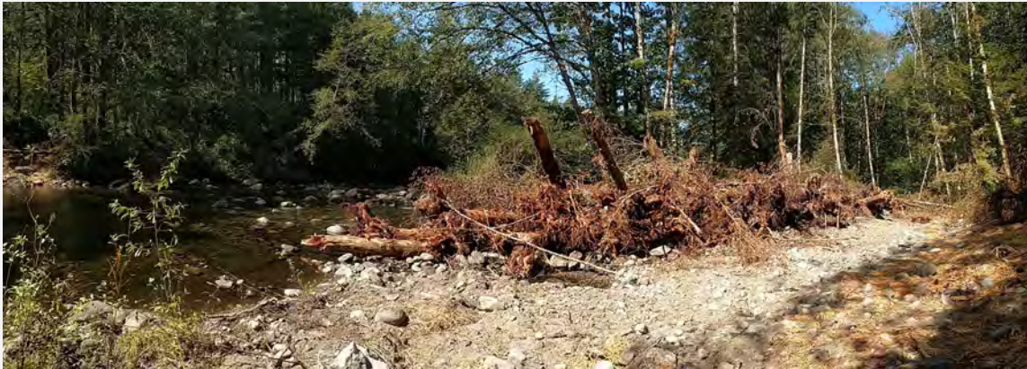
Figure 12. Zigzag Large 1A Channel Design; Apex Log Jam at the Downstream-most Berm Breach
