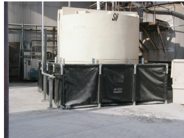
(d) Tank Secondary Containment Constructed with Flexible Liner System and External Support Framework.
