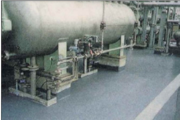
(a) Tank Vessel Showing CRC Applied to Floor. Containment Berm not Shown in Photo.
