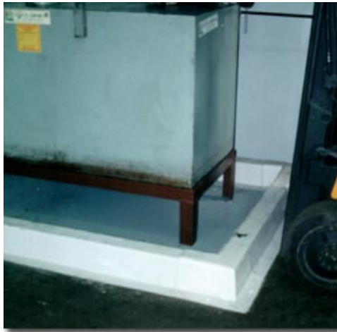
(a) Tank with Raised Curb and Floor Containment System Constructed from Chemical Resistant Materials
