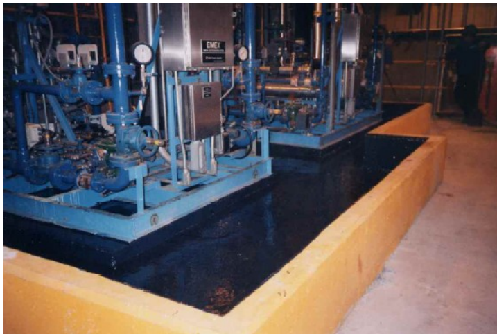
(c) General Installation showing Containment Berm and CRC on Interior of Containment
