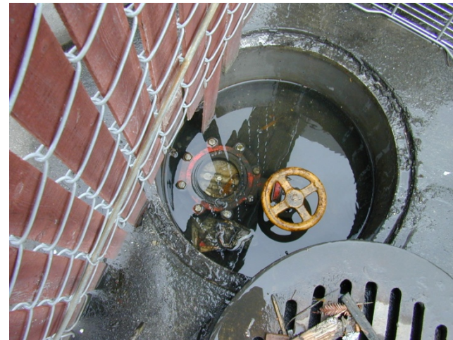
(d) Prefabricated Catch Basin Inserts ("Safe-Drains") with Butterfly Valve that can be Quickly Closed in Event of Spill and During Transfer Operations.
