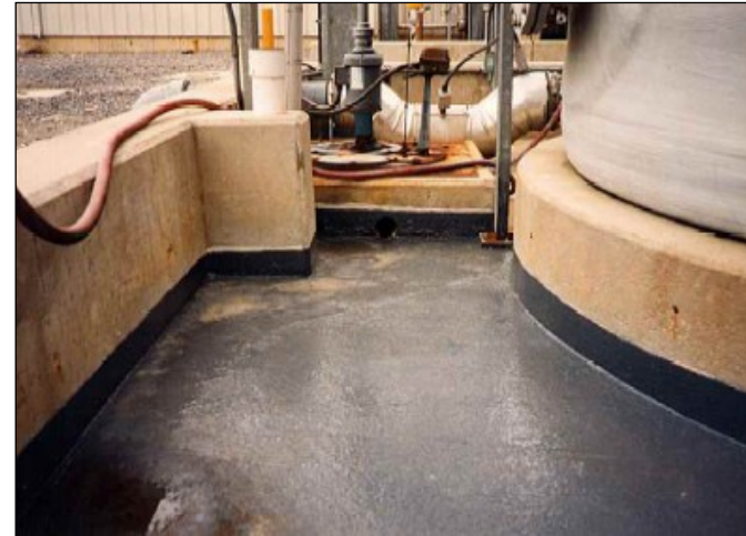
(b) Tank System shown with Perimeter Containment Berm and CRC
