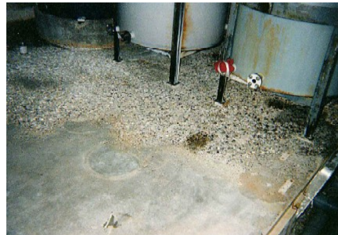
(d) Floor of Tank Containment System without CRC showing Exposed Aggregate from Continued Chemical Exposure
