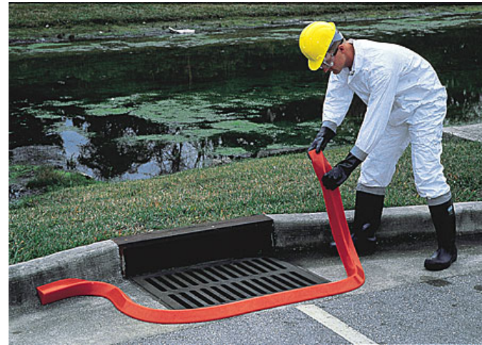
(b) Flexible Dike Materials can be Used to Isolate Drain Inlets.
