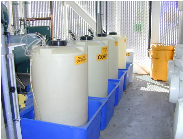
(c) Containment for Small Tanks/Larger Containers (Typical cost: $200-500)
