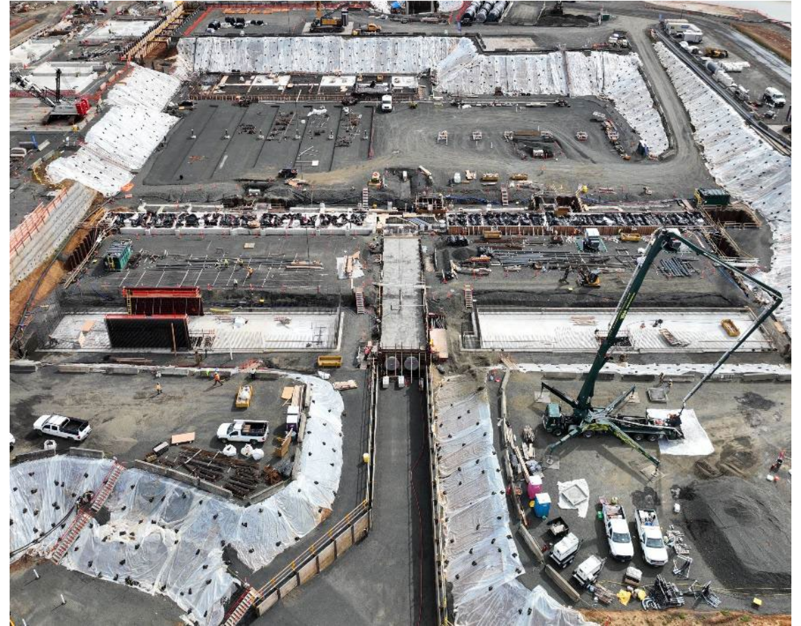
Filtration and sedimentation treatment basin construction (March 2026).
