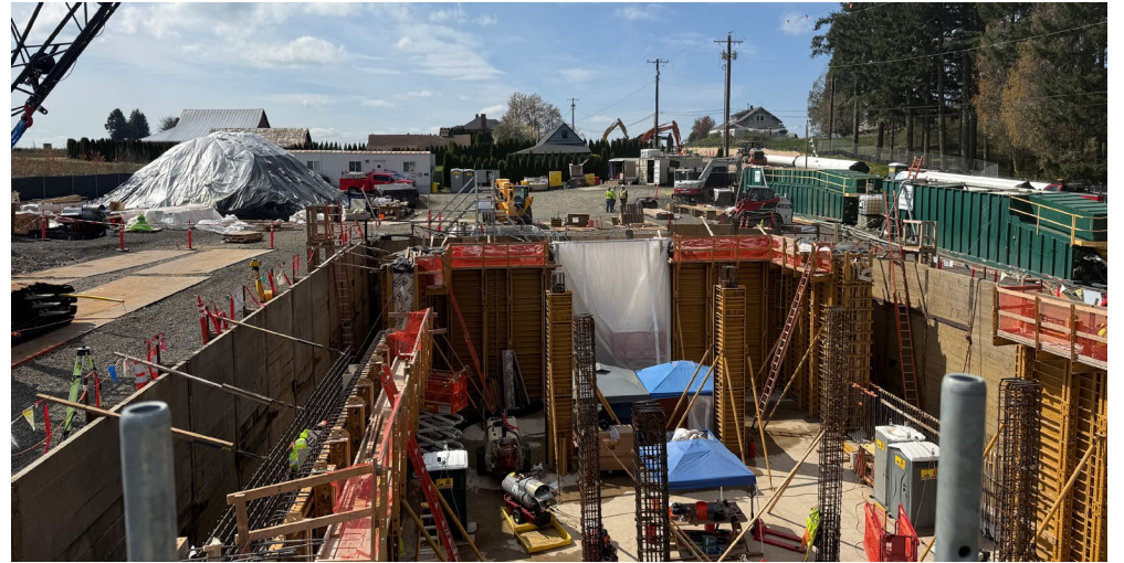
Finished water intertie construction (April 2026).
