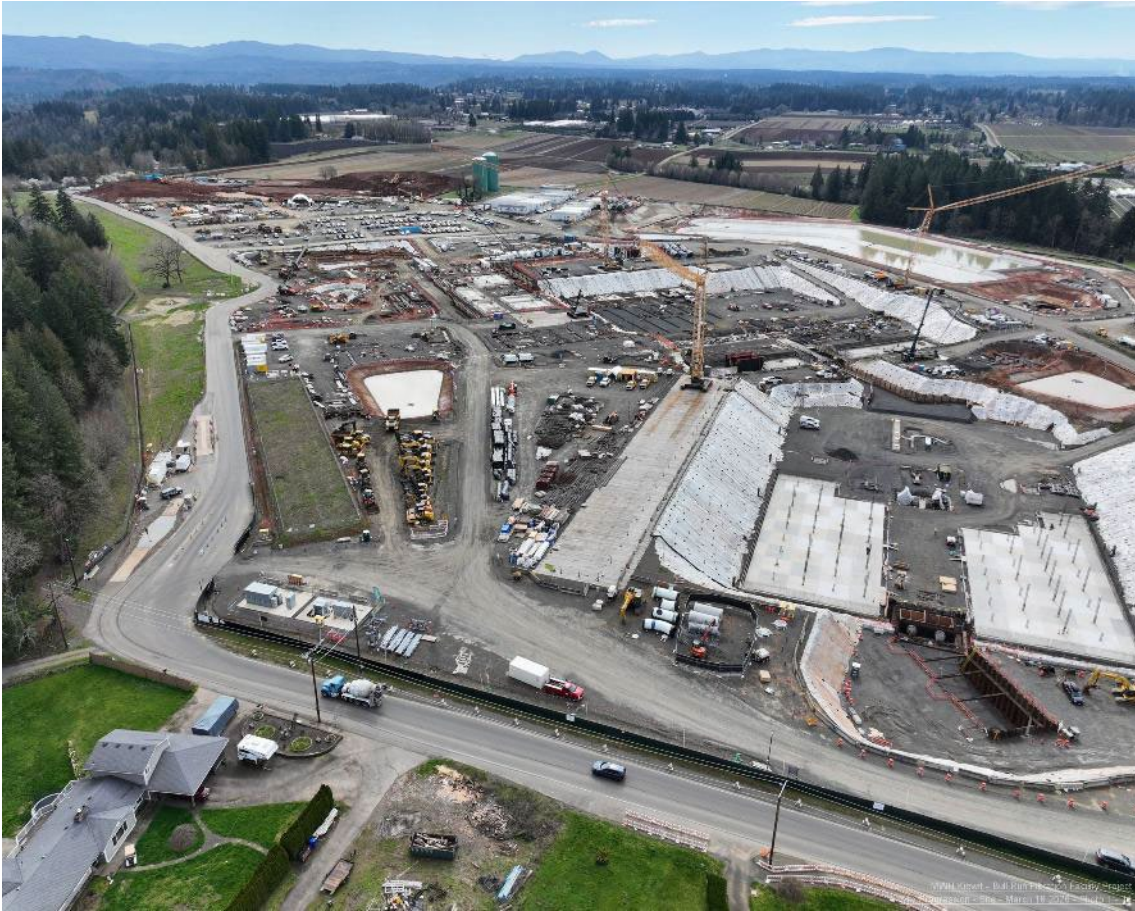
Looking south across facility construction site (March 2026).
