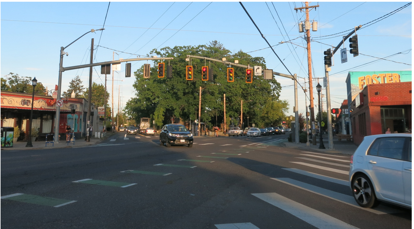
SE Holgate Boulevard intersects Foster Road at an angle. 63rd Avenue intersects SE Foster from the north and south on either sides of this intersection. There is also an alley on Holgate Boulevard 100' east of the curbs. This project made substantial changes to this intersection by removing a vehicle travel lane from each direction, adding continental crosswalks and crossbike pavement markings, changing signal operation, and adding a dedicated left turn lane to Foster Road.
