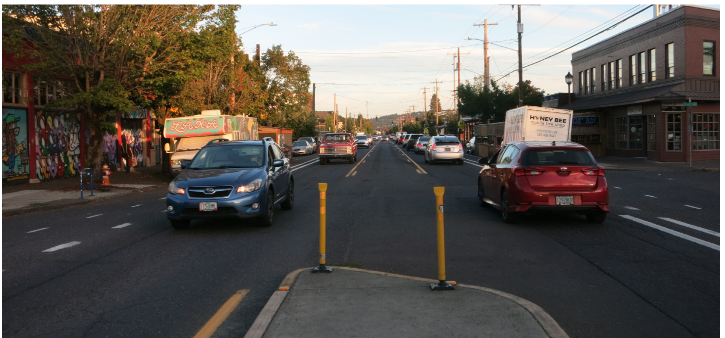
Median island at SE Foster Road & 65th Avenue
