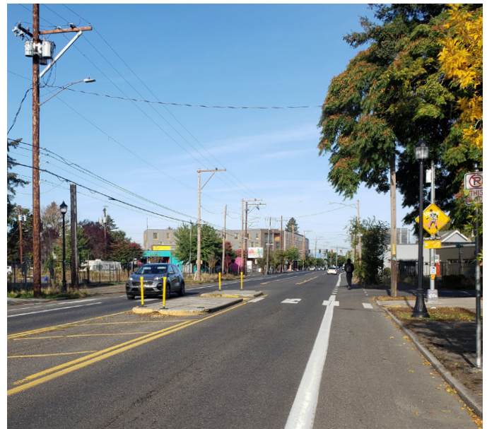
A flashing beacon and median refuge island on SE Foster Road at 74th Avenue.
