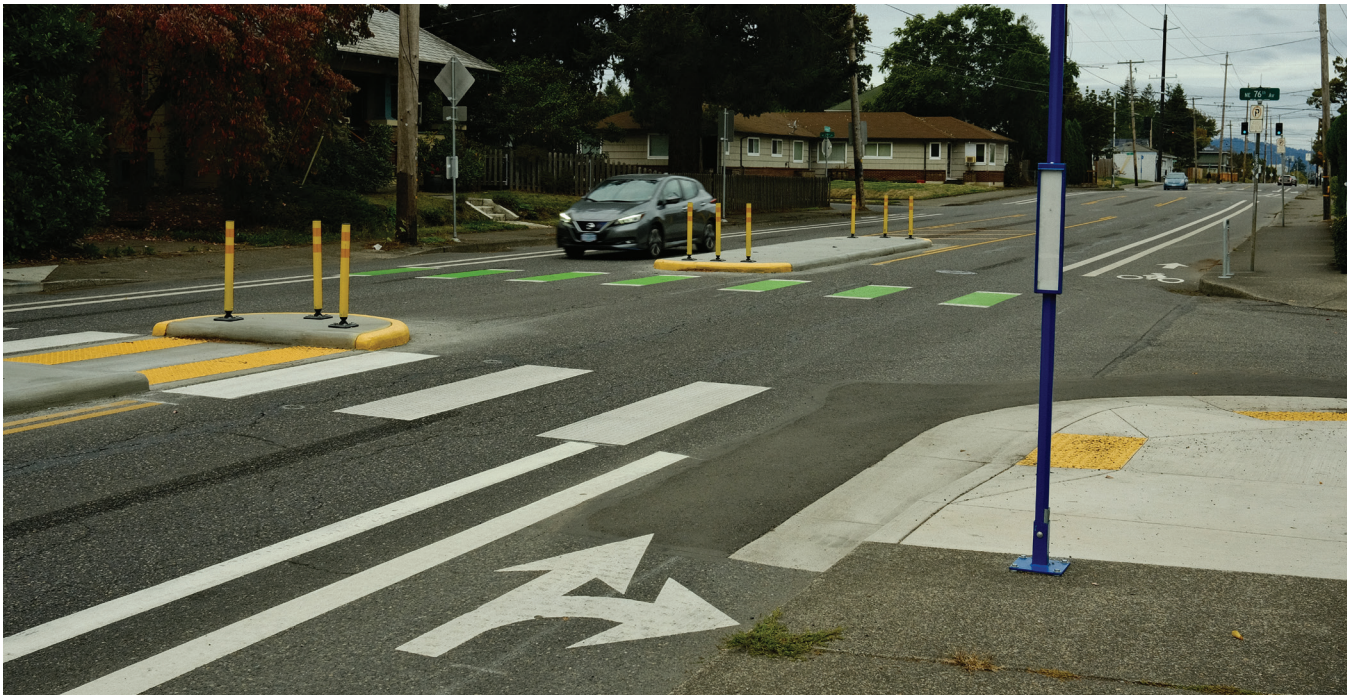
Figure 8. An improved intersection in Northeast Portland designed to shorten the crossing distance, slow driving speeds, and enhance safety for pedestrians and people biking.
