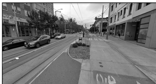
Figure 1 Before and after example of a road safety project: installation of two-way protected bike lanes and a road diet on Broadway in Seattle's Capitol Hill neighbourhood. Source: Google Street View.
