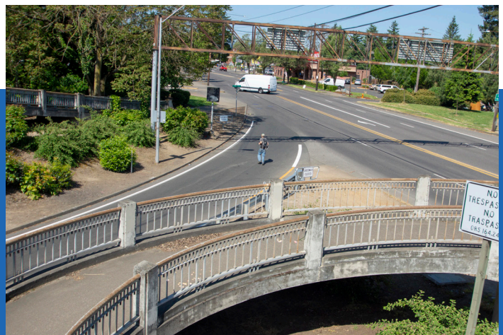
A pedestrian on N Lombard St crosses the I-5 on-ramp instead of using the pedestrian bridge.
