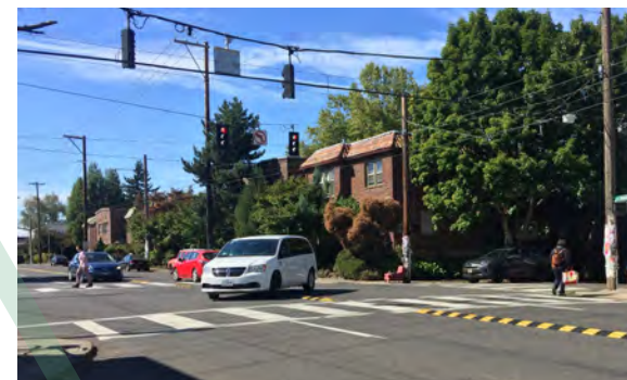
“Left-Turn” calming installed as part of a pilot project in Southeast Portland.
