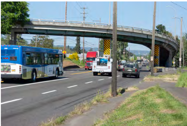
NE Columbia Blvd. Looking West Toward 33rd Ave Overpass
