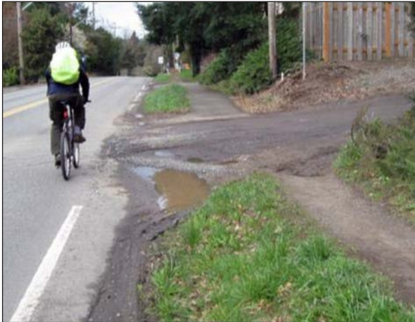
SW Baird Street intersection is typical of conditions in corridor—lack of formal bicycle, pedestrian and stormwater facilities.
