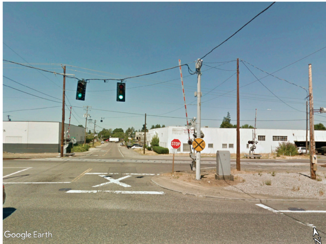
FIGURE 2. Active and passive treatments, heading north on NE 11th Avenue
