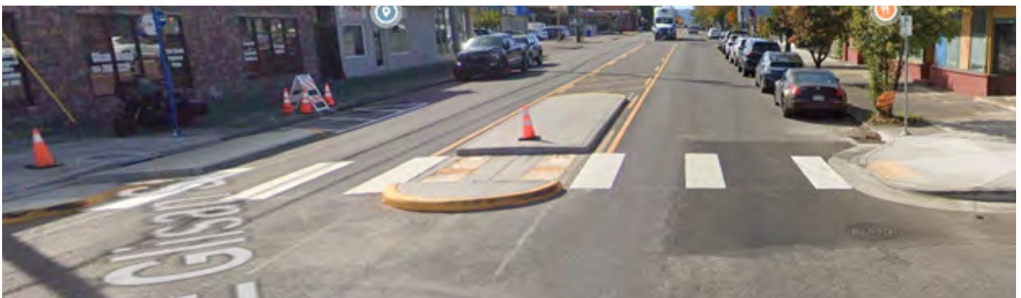
The crossing of NE Glisan Street at NE 80th Avenue before (left) and after (below). A marked crosswalk was added, along with a center pedestrian refuge island and curb extensions.
