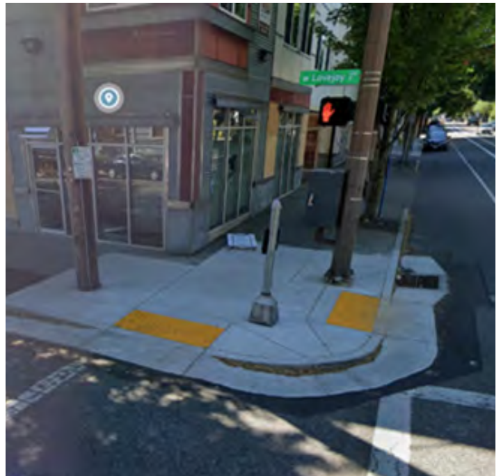
The SE corner of NW Lovejoy Street & NW 18th Avenue before (top) and after (bottom) the pedestrian signal was updated and new curb ramps were installed.
