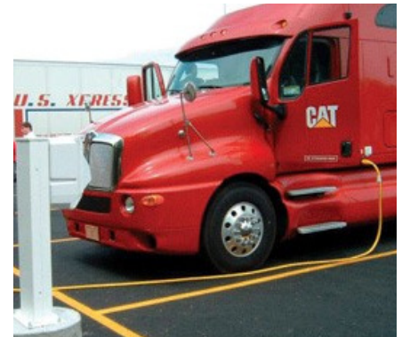
Picture 6.3: "Electric Hookup" A red freight truck connected to an electric vehicle charger. The charging system is white, the charging cord is yellow. [Source: unknown]
