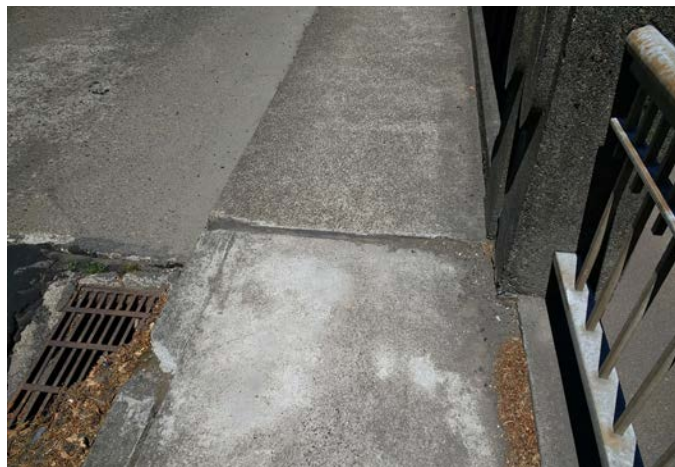
The sidewalk on the bridge is less than four feet wide, creating safety concerns and mobility challenges for people using mobility devices.
