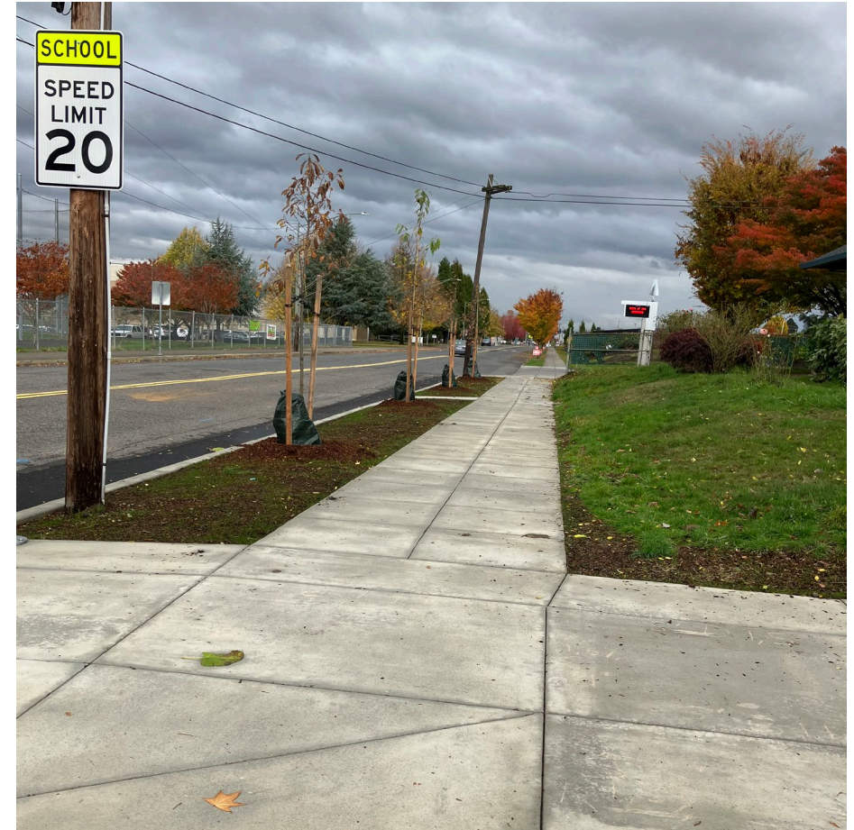
Completed sidewalk on NE Shaver St
