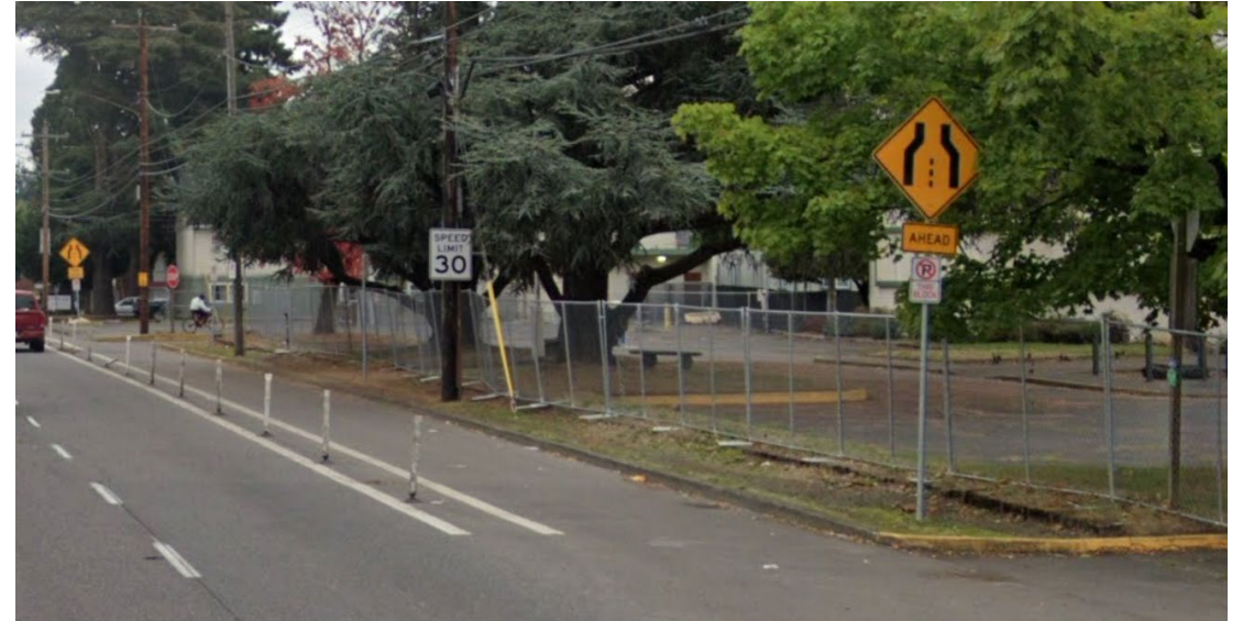
Missing sidewalk on NE Glisan St east of 122 nd Ave
