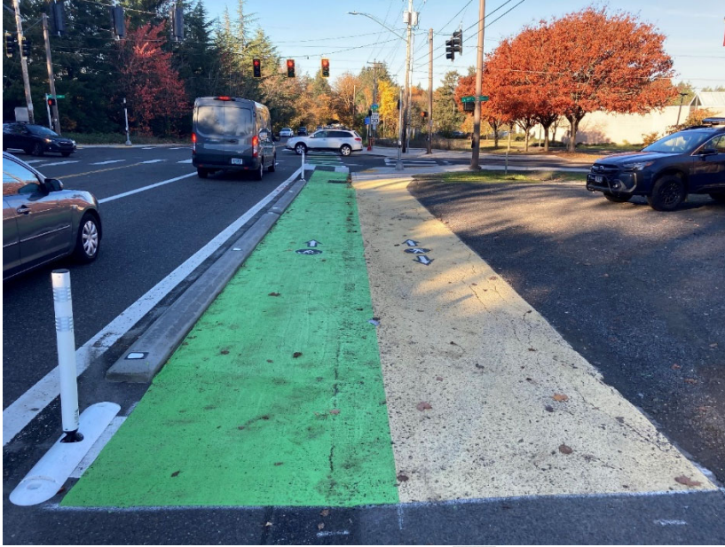
Figure 2 - Alternative walkway and bikeway on SW Multnomah Boulevard between 37th and 40th Avenues, using concrete separators and green and yellow paint.
