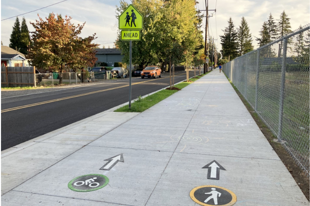
Figure 3 - A concrete multi-use path was completed on SE 174th Avenue between Stark and Main streets, serving Alder Elementary School in the Reynolds School District.
