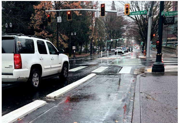
Image: Concrete separators in bike lane buffer preventing vehicular turn incursion into bike lane at an intersection
