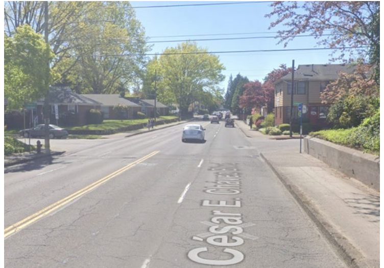
Image: Existing conditions, looking south down SE Cesar E Chavez Boulevard toward the intersection with Francis Street
