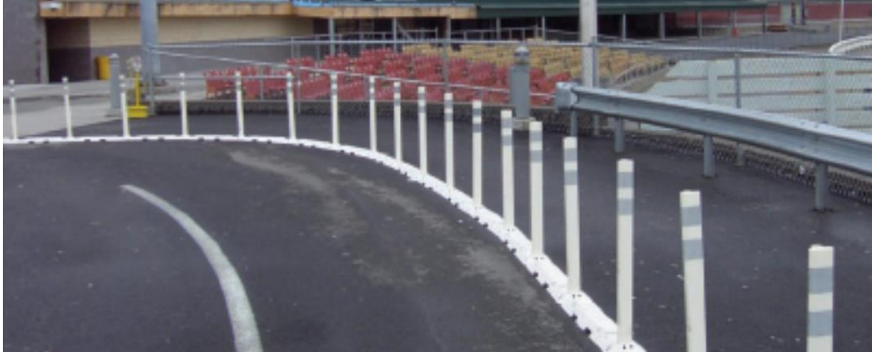
Figure 4.7 Temporary Curb Installation as Detectable Edging
