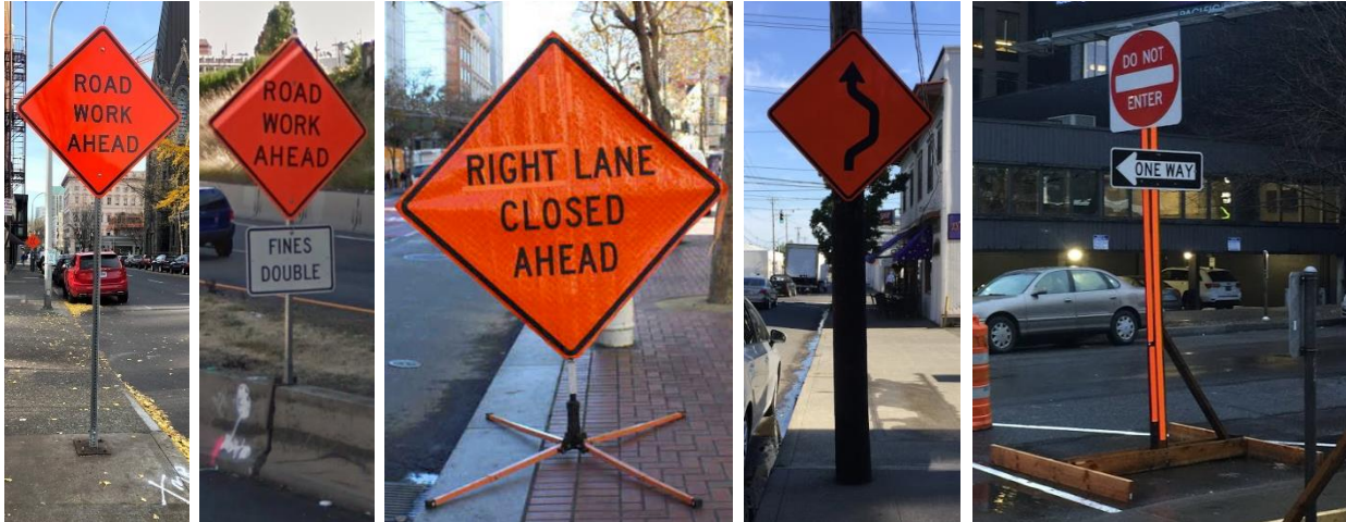
Figure 4.1 Typical Sign Supports
