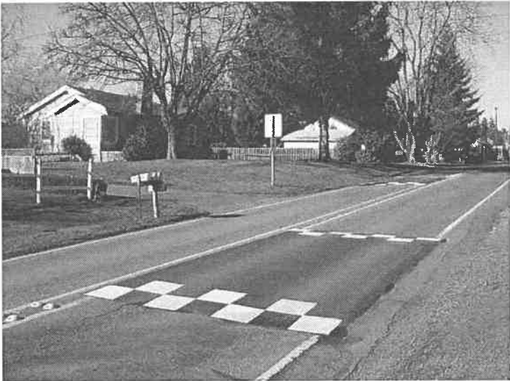
Photo 4. Beaverton Offset Speed Hump Centerline RRPMs.
