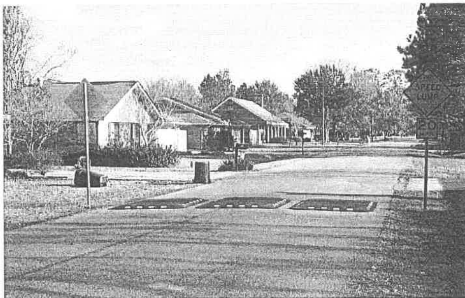
Photo 1. Speed Cushion, Lafayette, LA.
