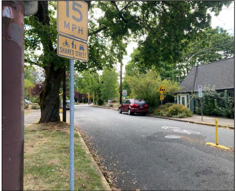
Image shows multiple signs installed along NE 53rd Ave.
