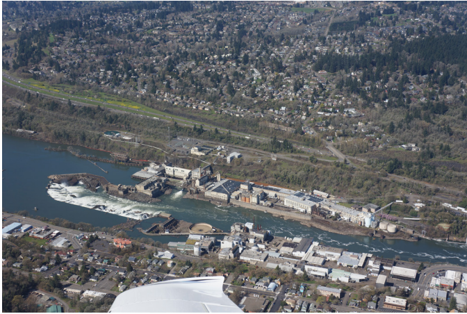
Photo: Aerial view of Willamette Falls Locks
