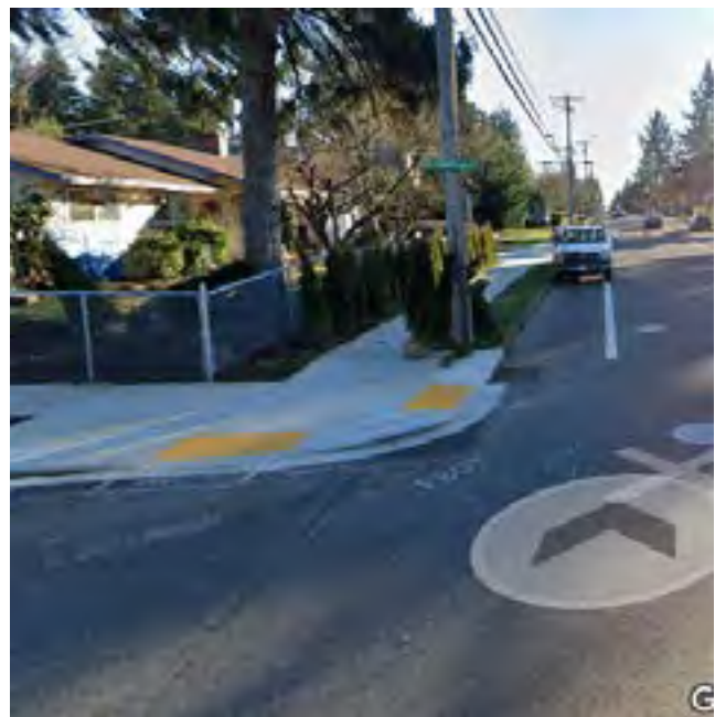
This is the corner of SE 130th & Morrison. Sidewalk was added beyond the corner for approximately 150'. Source: Google Maps
