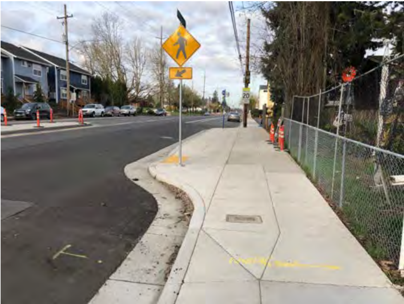
This is a transit stop #3209 at NE Killingsworth & 57th where the sidewalk was extended to allow the bus to get directly next to the curb for boarding and exiting the vehicle. Source: TriMet.
