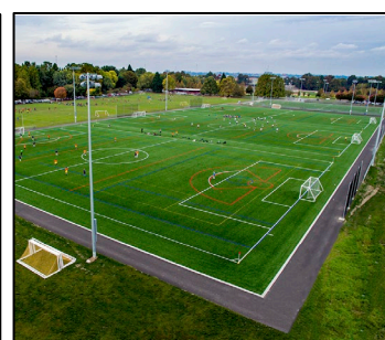
Improvements at Delta Park
