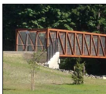
Pier/Chimney Park Bridge
