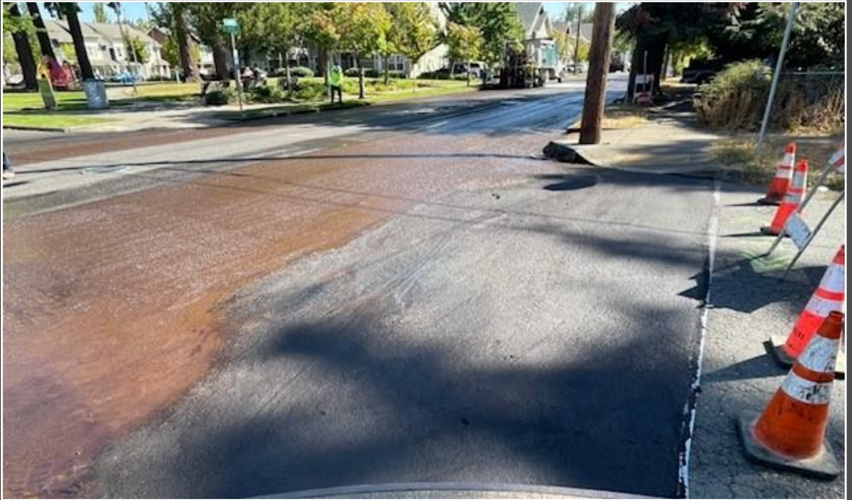
Slurry Seal
