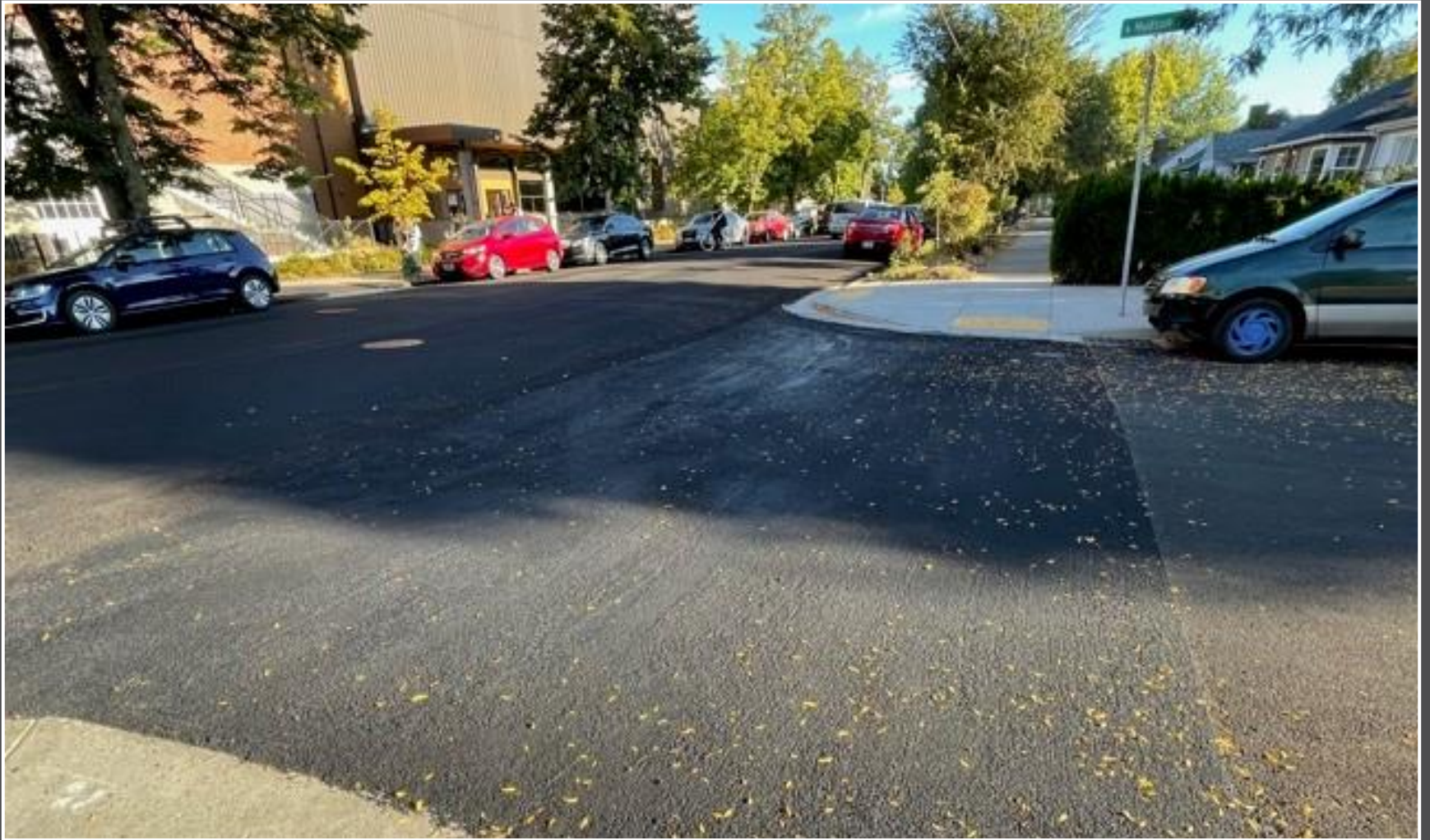
Microsurfacing – N. Ida (after)
