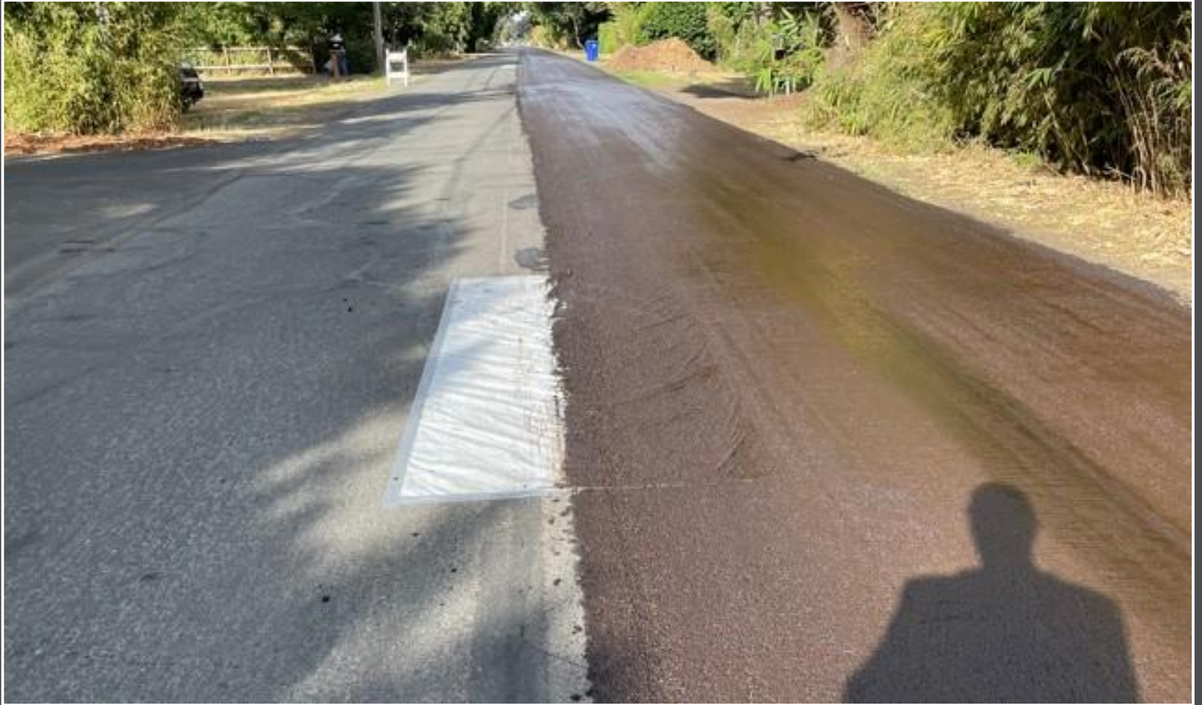
Slurry Seal (N Houghton)
