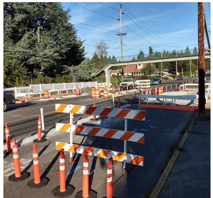
Crossing in front of Menlo Park Elementary School under construction.
