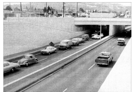
Powell under crossing at 17 th Ave, 1979. City of Portland Archives
