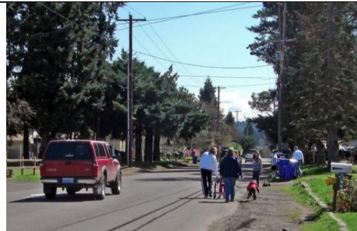
2. Paved street without curbs
