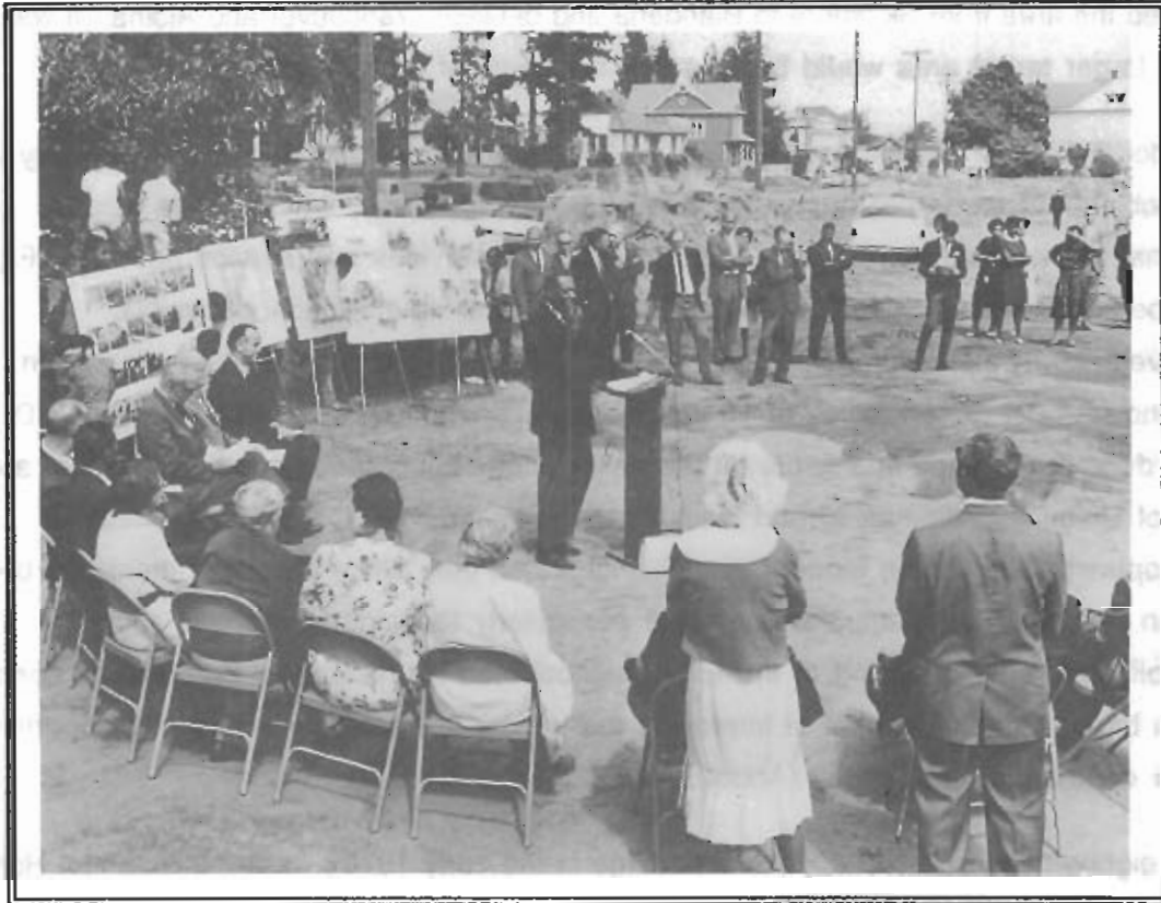
Groundbreaking for Unthank Park-1967 (OHS)
