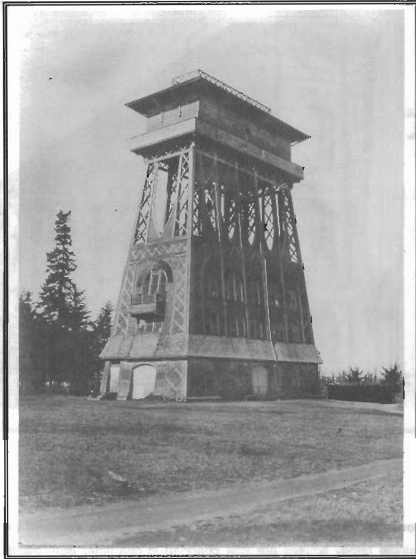
Piedmont Water Tank ca 1899 (OHS)
