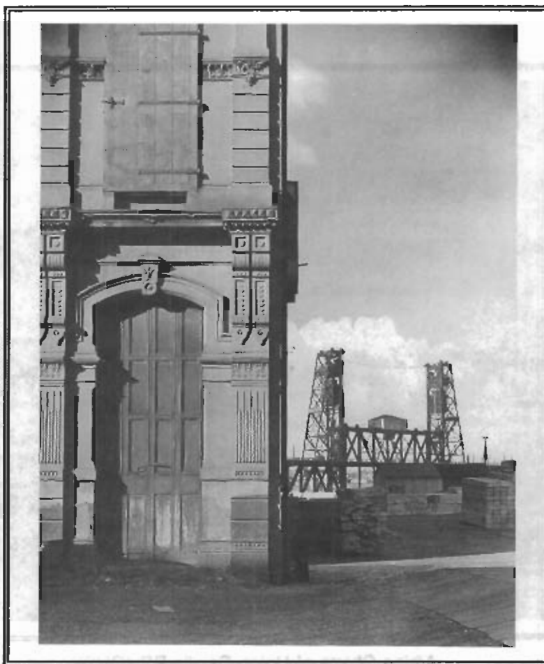
Steel Bridge-Minor White-1940 (OHS)
