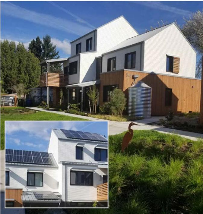
Striving towards net zero with features that include photovoltaic panels on all south-facing roofs, triple-paned windows to limit the amount of hot and cold air and cisterns for collecting rainwater.
