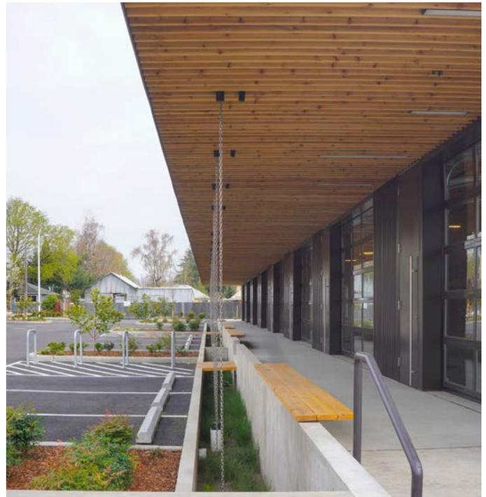
Collecting stormwater runoff from parking areas and rooftops in a visible and compelling way.
