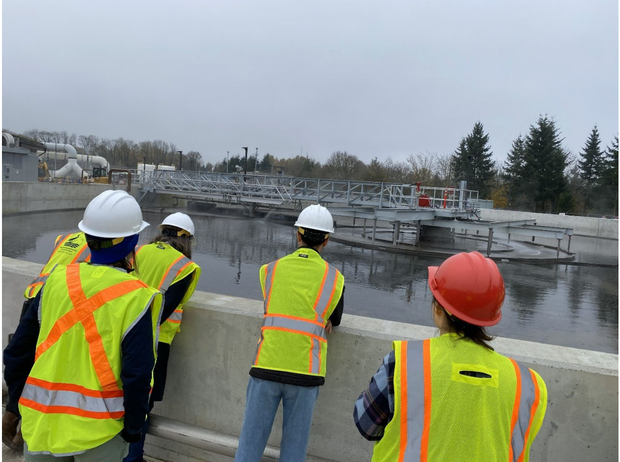
Figure 3: PUB members and City staff viewing the new secondary clarifiers that were completed December 2024 - part of STEP improvements increasing their biological treatment capacity and resiliency
