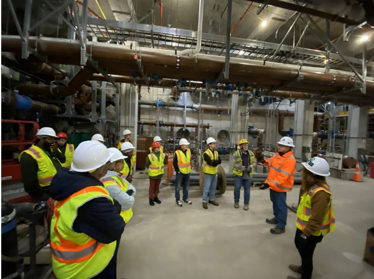
Figure 5: PUB Members, City staff, & Contractor touring the biosolids processing facility. Pictured from left to right: Darrel Bobb, Anthony Locke, Kyle Chipman, Lauren Rosenkranz, Cormac Burke, Ri Sandel, Construction manager, Brian Gomolski.
