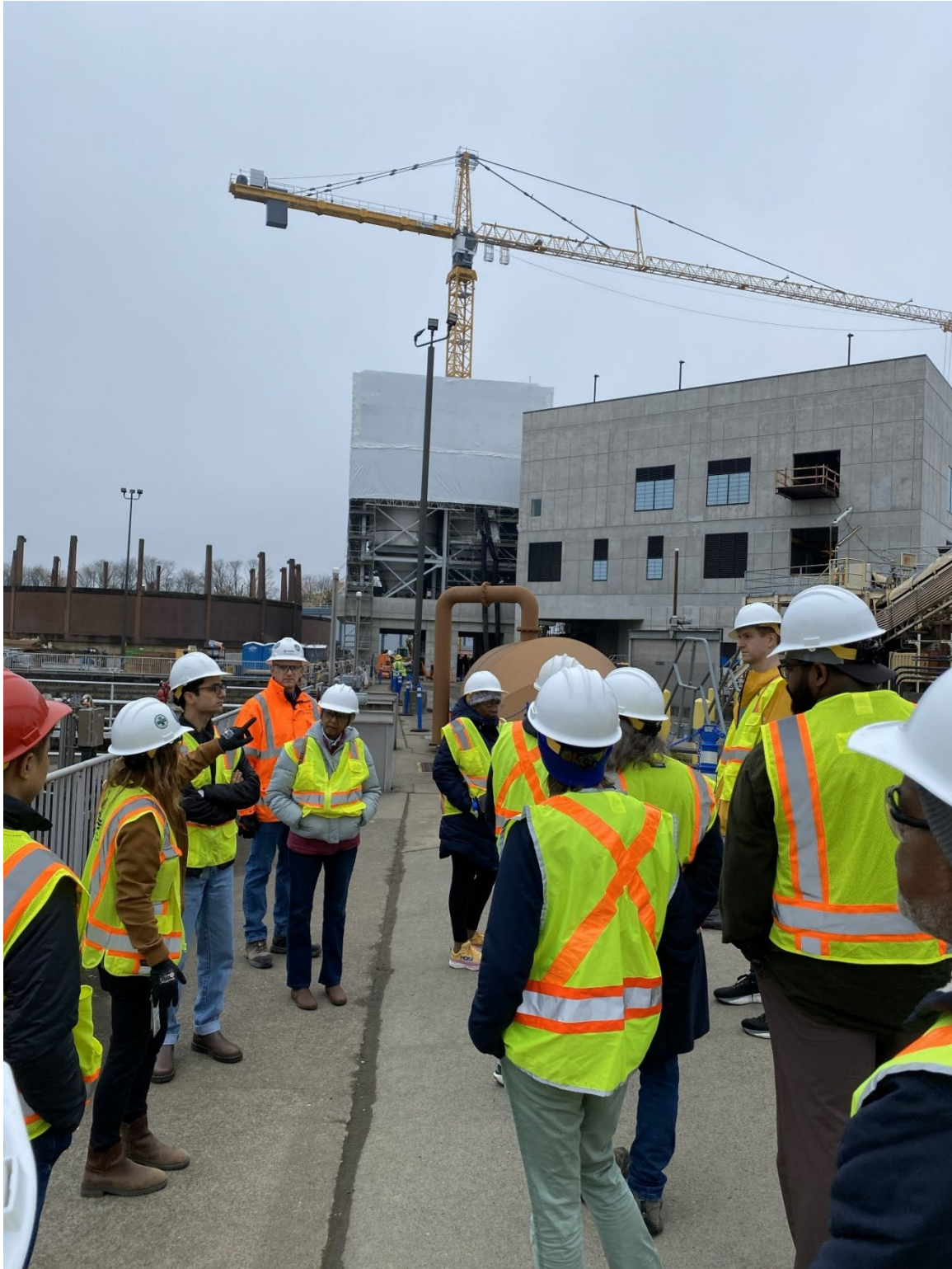
Figure 4: City staff (Muriel Gueissez-Teufel) describing updates in progress to PUB members viewing ongoing construction the new biosolids processing facility that is replacing the existing building that is failing. Pictured: Ri Sandel, Stantec contractor, Antoinette Gervais, Lorraine Wilson.
