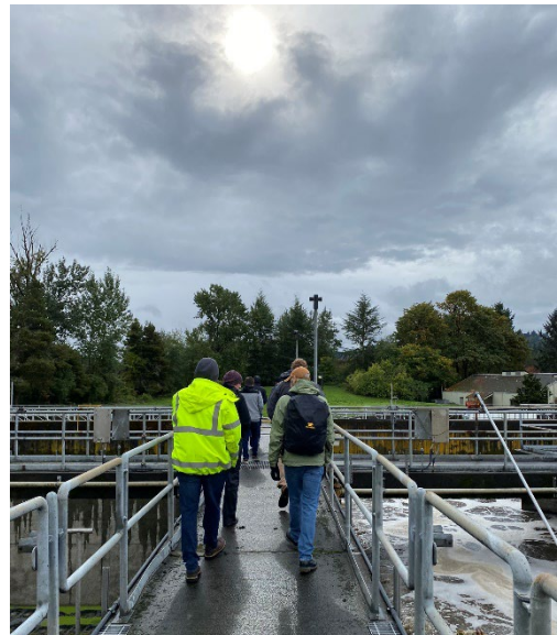
Figure 4- PUB viewing/walking over aeration basins at Tryon Creek Treatment Plant, October 2023
