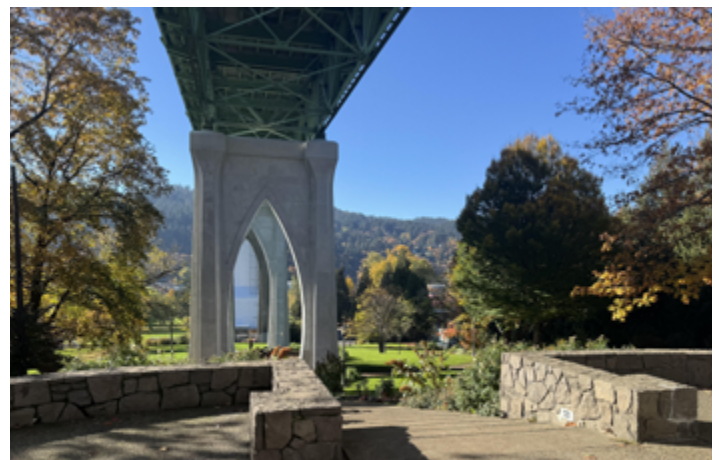
Staircase and Deck in Cathedral Park
