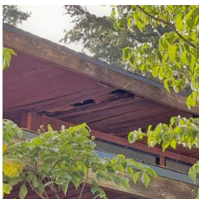
WOOD DETERIORATION AT OVERHANG
