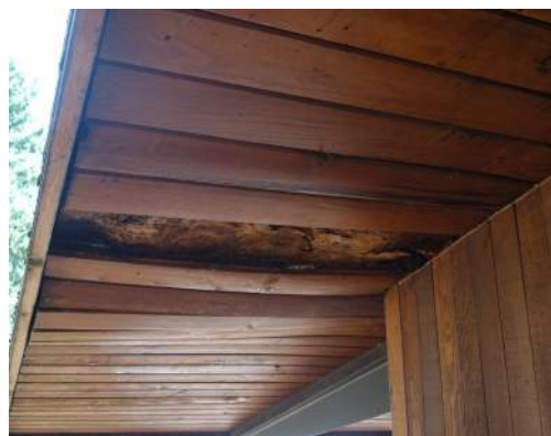
WOOD DETERIORATION AT OVERHANG
