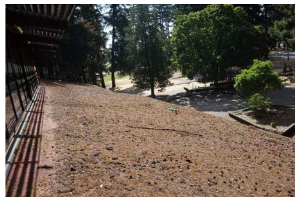
DEBRIS AND MOSS BUILD-UP ON ROOF
