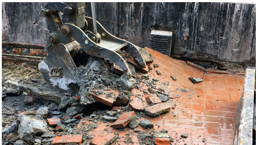
REMOVING THE UPPER DECK AT PIONEER COURTHOUSE SQUARE
