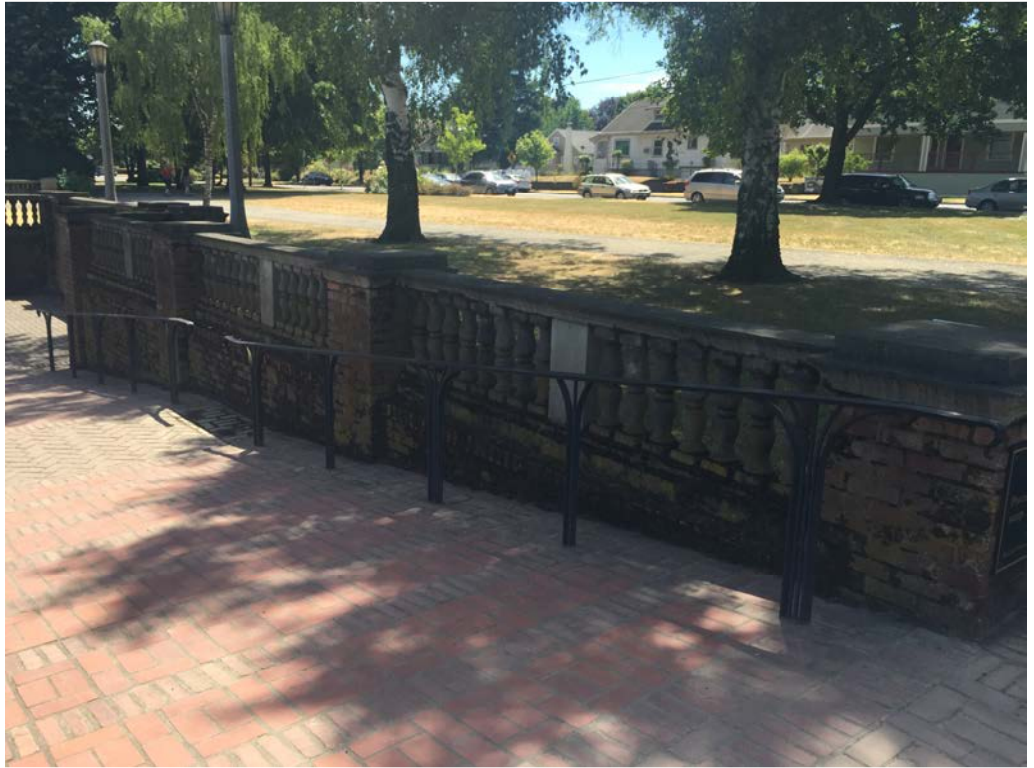
Heavy accumulation of moss on vertical wall below balustrade; moss must first be removed with a wire brush to prevent accelerated decay and to assess relative need for repoint.
