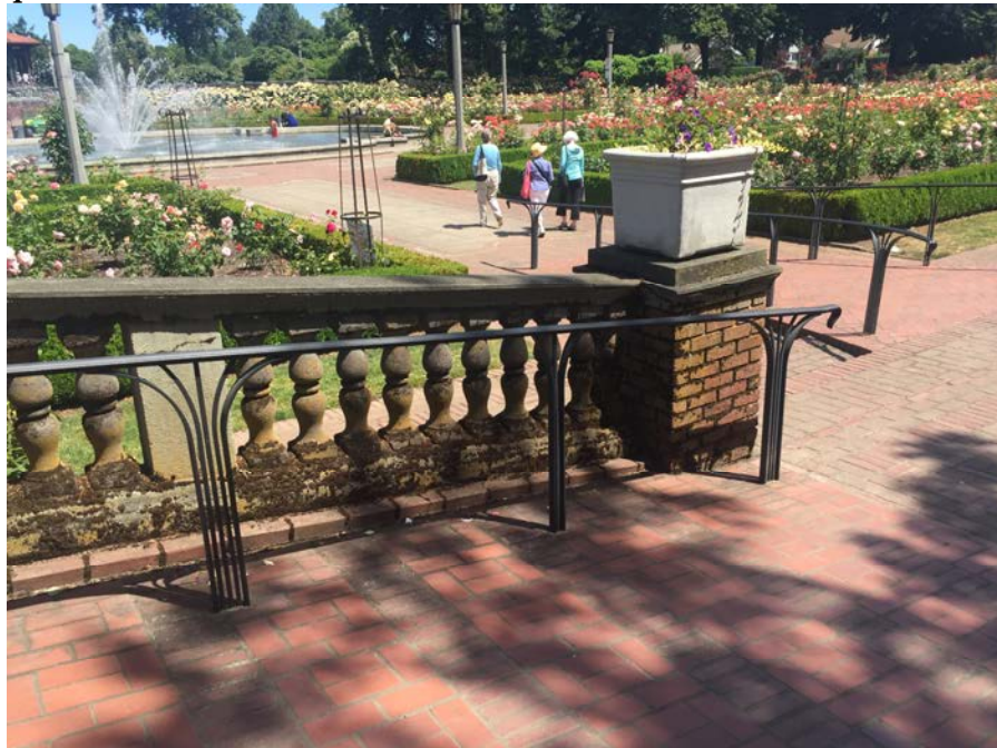
Balustrade with heavy accumulation of moss. Cracks in base of banister are evident by linear distribution of moss. Moss must first be removed in order to assess damage and make repairs.
