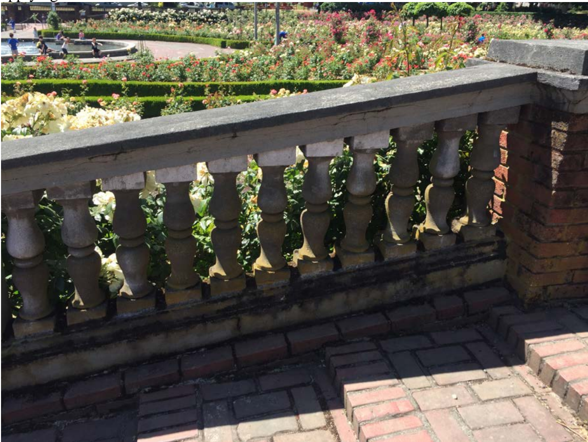
Bannister with various small cracks, accumulation of moss.
