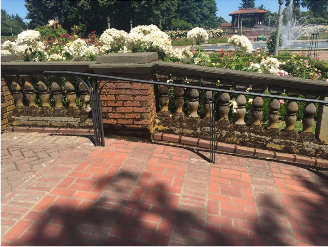
Balustrade with heavy accumulation of moss. Cracks in base of banister are evident by linear distribution of moss. Moss must first be removed in order to assess damage and make repairs.
