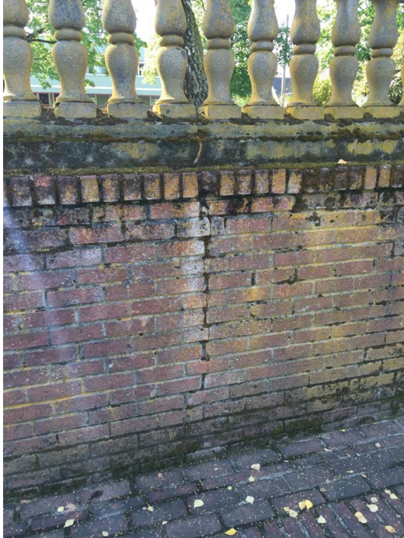
Brick wall below cast concrete balustrade. Note long vertical crack infilling with moss and wider at the top than bottom. Crack extends to coping above.
