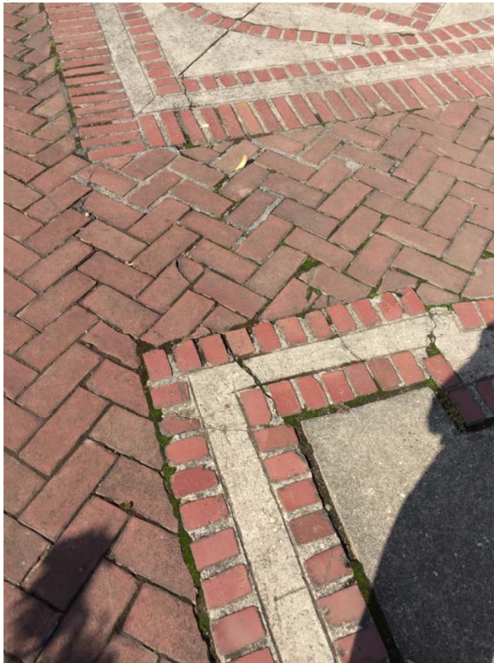
Flatwork exhibiting fissures between herringbone brick and concrete border
