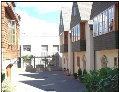
Jake's Run townhouses, Northwest Portland
