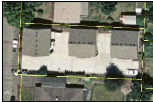
Multidwelling projects with 20'-wide driveways meeting the minimum dimensions required by Title 17.
