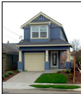
Left: While similar in basic form to other narrow houses, this house's porch extends beyond the usual 15'-wide dimension, helping to counter this housing type's narrow, vertical appearance and providing a better contextual fit with nearby bungalows
