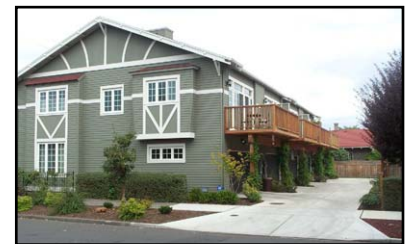
Rowhouses with cantilevered rear balconies over rear alley.
