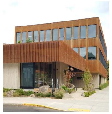
Sourcing regionally harvested and locally manufactured materials, including Cross-Laminated Timber (CLT), weathering steel, Oregon juniper, cedar, and river rock and boulders. **Belmont**, SE Belmont and SE 14th
