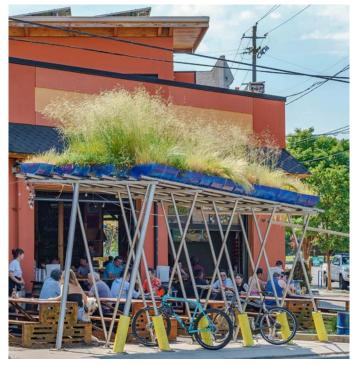
Designing stomwater runoff systems to be multi-functional. This installation manages stormwater, covers bicycle parking, and serves as public art. **Dekum**, NE Dekum and NE Durham
