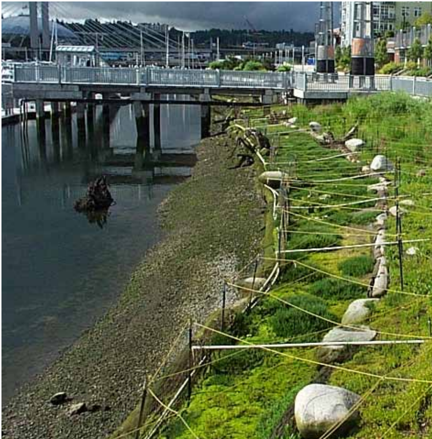
This photo shows a bank in Tacoma, Washington, where the viewpoint is cantilevered over the bank, minimizing impacts to a continuous habitat corridor below.
