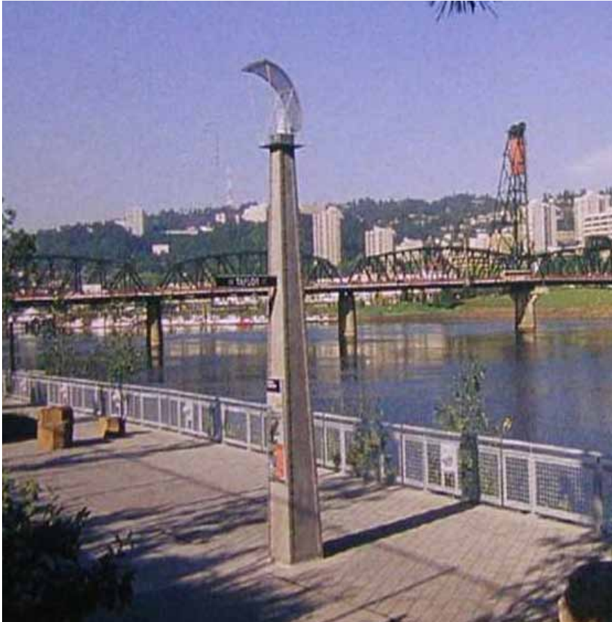
Light fixtures like this one on the Eastbank Esplanade offer focussed light from the directional piece onto the ground below. In addition, the hood component catches excess light from the fixture and spreads it indirectly over a slightly greater area, increasing efficiency of the fixture.
