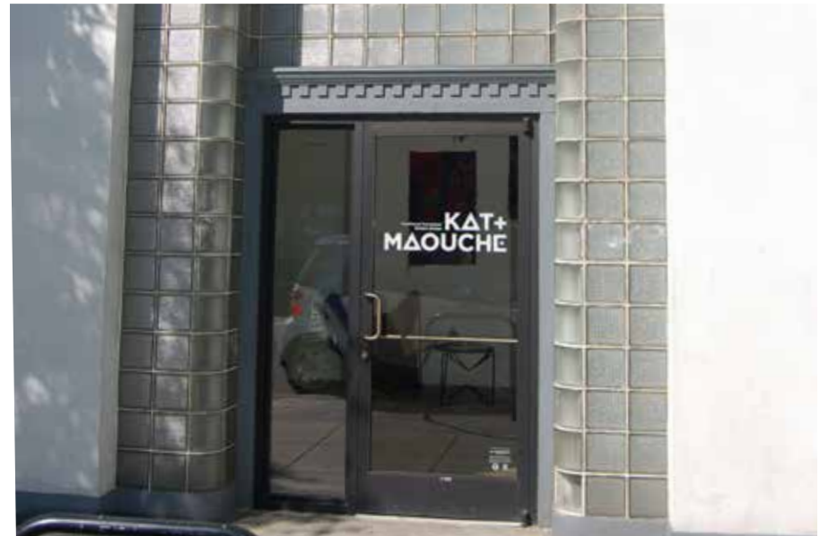
This curved-wall glass block entry is a character-defining feature of the building. It shows the Moderne sub-style detailing used on this 20th Century Commercial style building on NW 4th Avenue.
