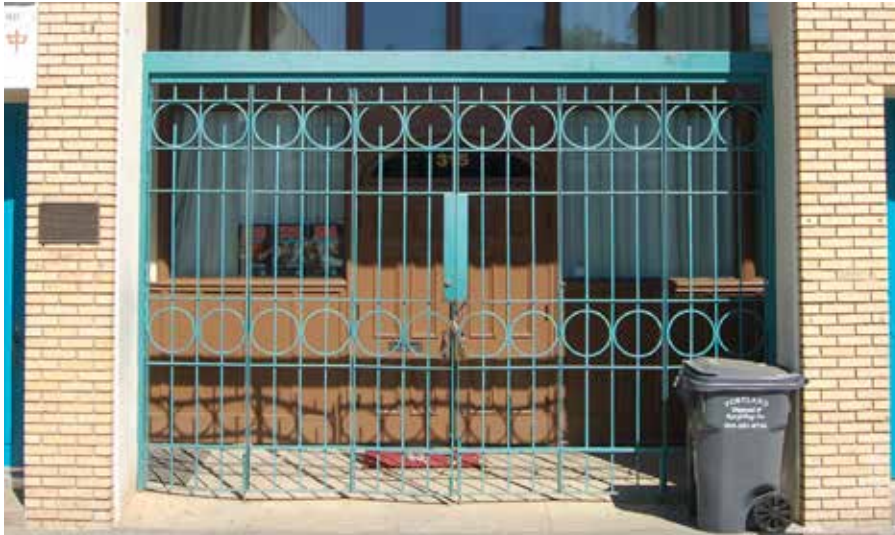
The folding security gate at the Chinese Consolidated Benevolent Association was designed to fit its opening with minimal impact to the storefront and adds Chinese decorative detail to the entry.
