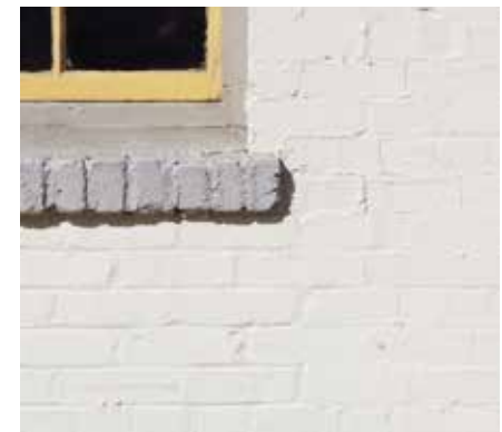
Avoid painting brick, but if existing brick is already fully painted, as at the Columbia River Ship Supply building, repainting is acceptable.
