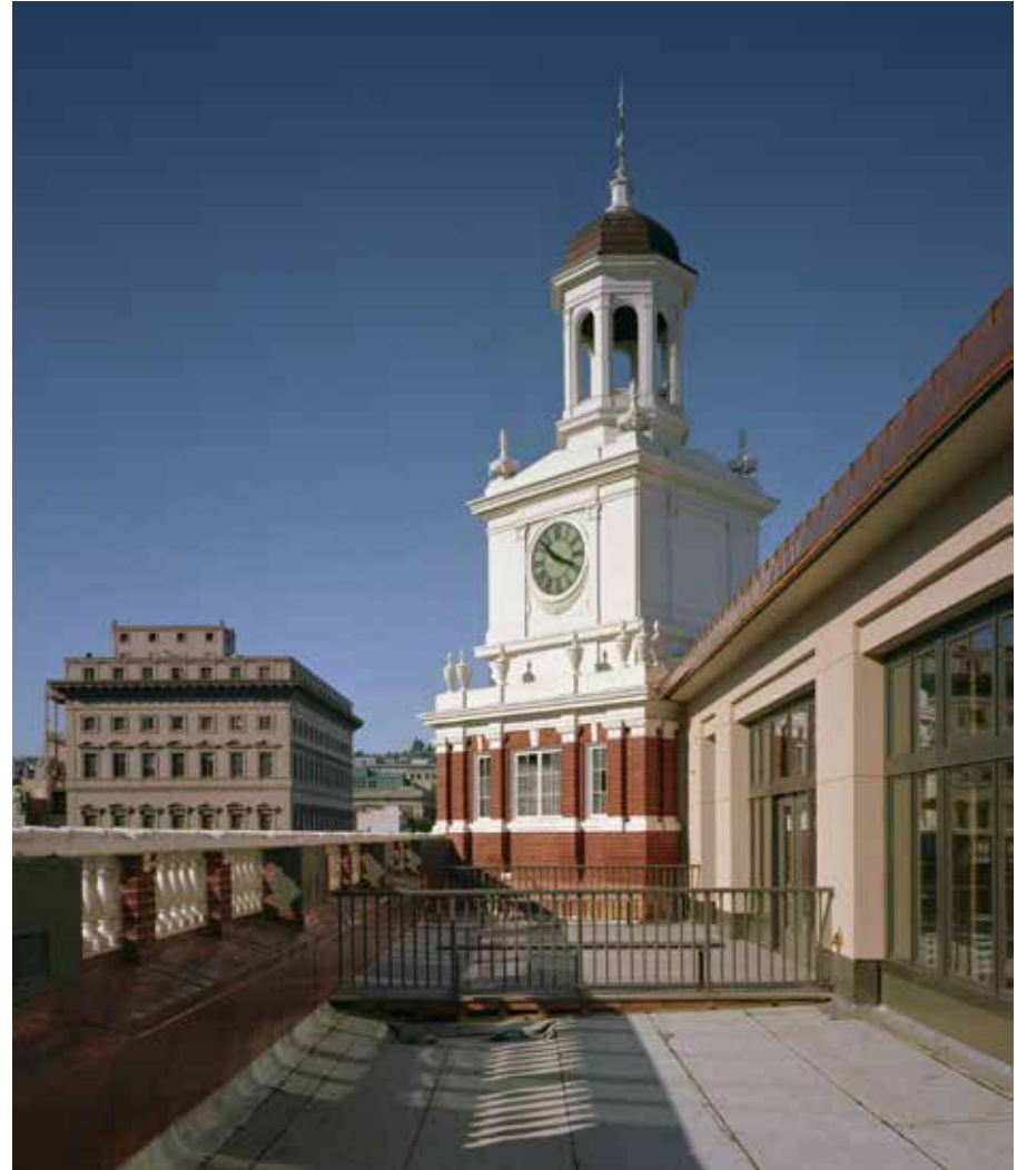
The added penthouse on the historic Telegram Building on SW Washington Street is set back from the façade and is almost invisible from the street.
