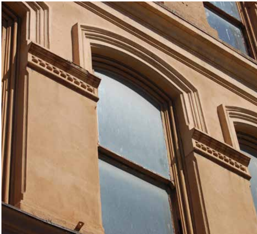
The predominant wall finish at the Sinnott House is a smooth concrete stucco.
