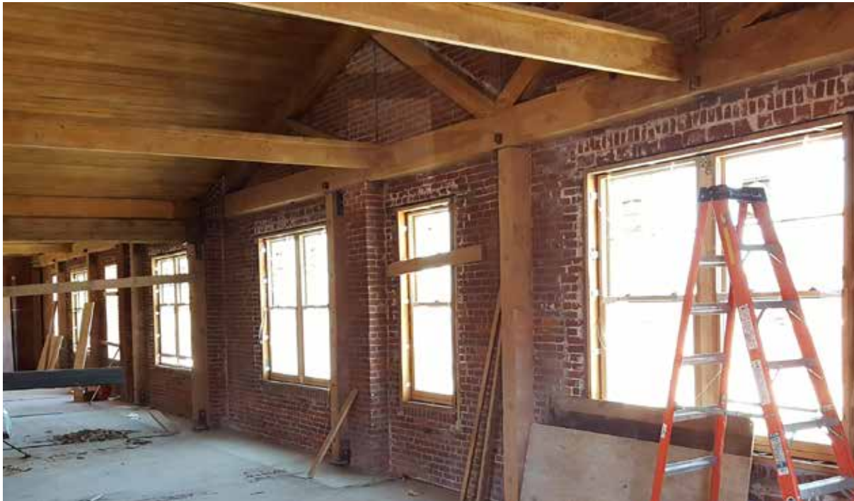
The Overland Warehouse seismic retrofit solution was able to retain existing heavy timber and add metal reinforcements at the timber joints and between the brick walls and the timbers. Courtesy of Emerick Architects.
