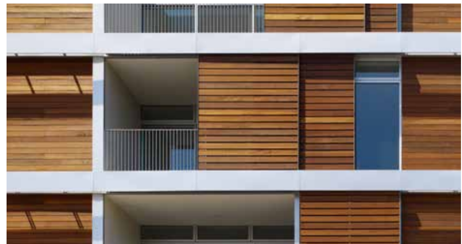
The Hancock Lofts in Malibu, California, uses sliding wood shutters, a sunshading device which also recalls traditional Japanese screens. Courtesy of ericstaudenmeier.com.
