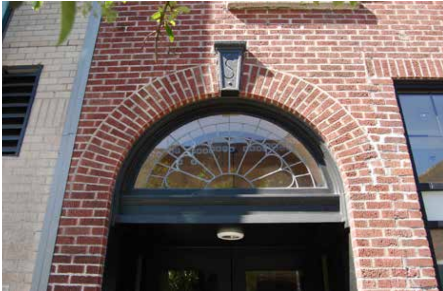
The Union Gospel Mission Building brickwork has highly contrasting mortar joints.
