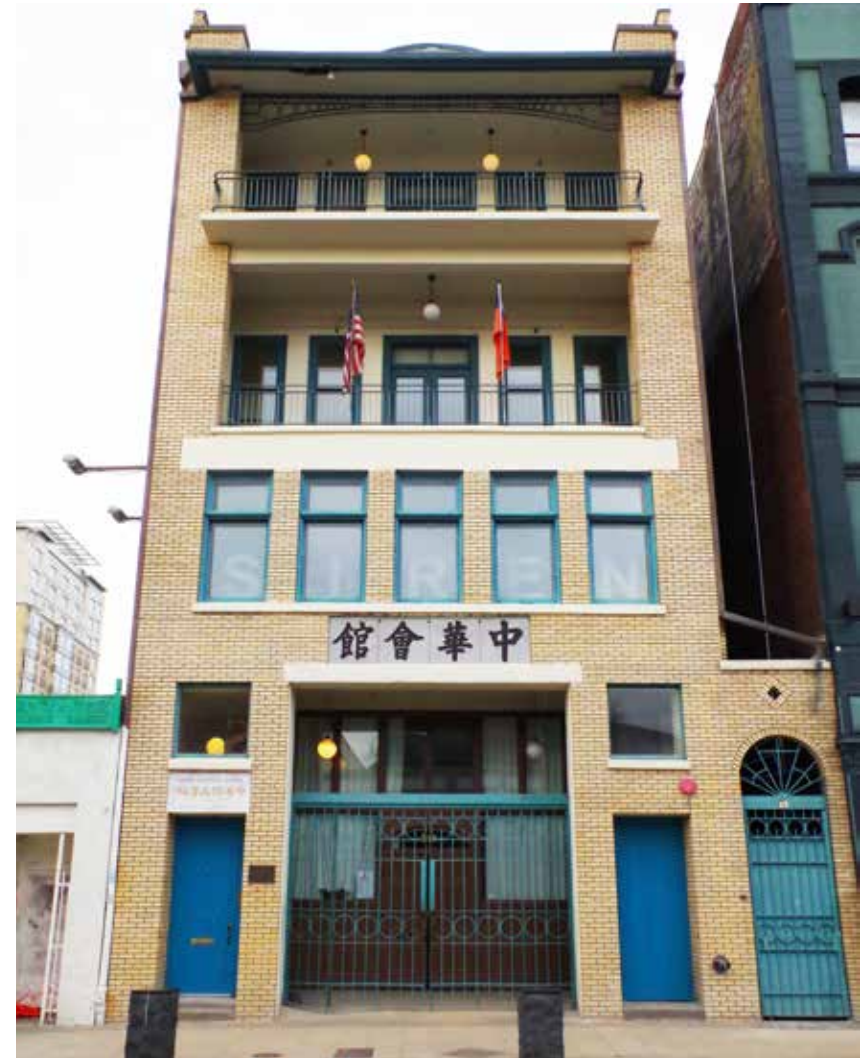
The Chinese Consolidated Benevolent Association Building was constructed in 1911 and is a good example of a 20th Century Commercial style building with Chinese-influenced details such as the decorative metalwork, recessed balconies, hipped tiled roof projection at the cornice, and expressed lintels, as well as added embellishments such as signs, rich colors, and hanging flags.
