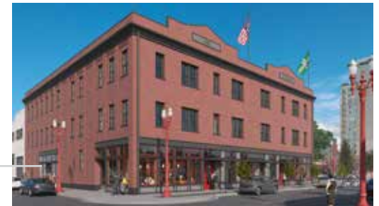
The Overland Warehouse at 4th and Davis was rehabilitated to retain the historic pattern of window and storefront openings. Historic materials were repaired and, where necessary, replaced with materials in keeping with the original. Images courtesy Emerick Architects.
