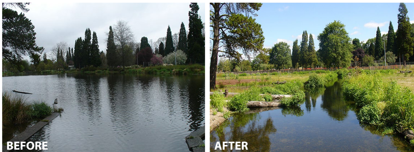
Crystal Springs Creek before (left) the removal of a large inline pond in Westmoreland Park and after (right) the City implemented the project to restore the natural stream channel. The pond added heat to Crystal Springs Creek, increasing water temperatures by 2-4°C. These substantial increases in temperature are no longer observed.
