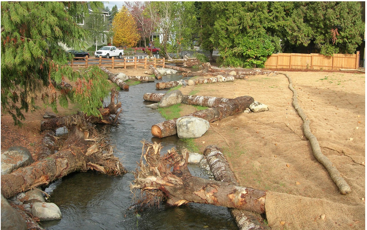
Restoration of Crystal Springs Creek between SE Tenino Street and SE Umatilla Street. Two culverts were replaced to provide fish passage and large wood and boulders were added to the channel to provide habitat.
