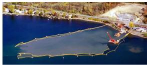
Turbidity curtains are designed and selected for specific flow conditions. For sites with flow velocities or currents greater than 5 feet per second, a qualified engineer and product manufacturer must approve of the use.
