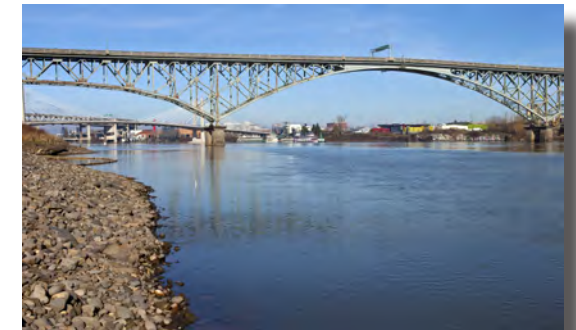
Ross Island Bridge
