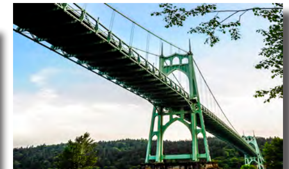
St. Johns Bridge
